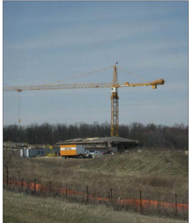
Image 7-3: Water Reclamation Facility; Source: BHC
