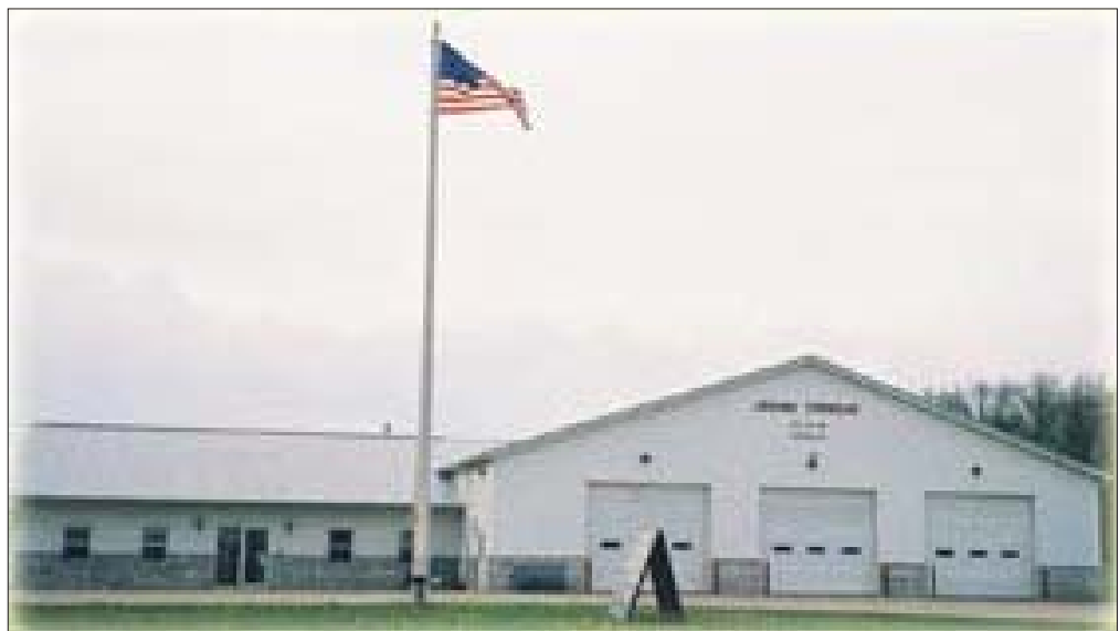
Image 7-5: Fire Station; JT Website
